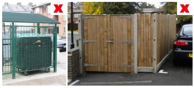
1. Inadequate screening. 2. Unacceptable - Timber frame vulnerable to impacts.
