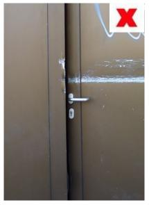
5, 6 and 7—those doors are not constructed of robust materials and have become damaged as a result.
