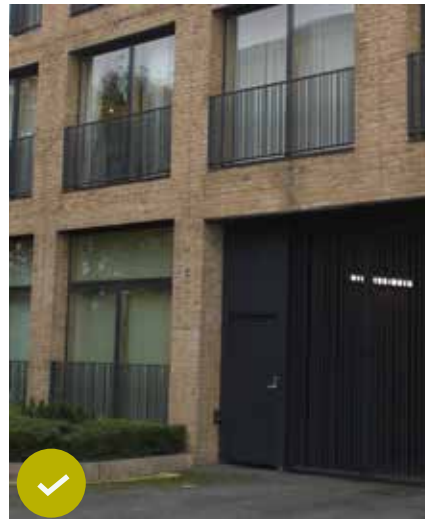
Well designed vehicular entrance
