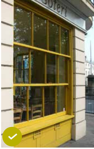
Triple sash window
