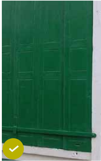
Traditional timber shutter
