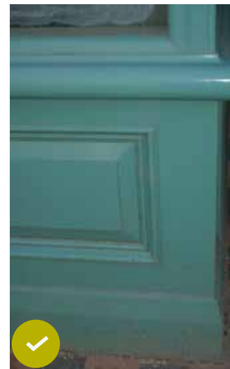
Timber stall riser
