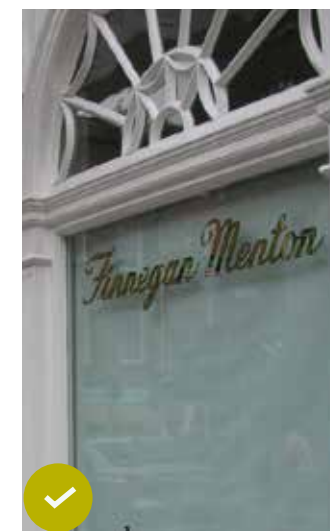
Internal blinds deter smash and grab
