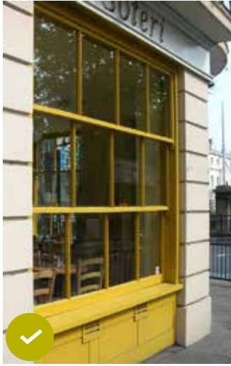
Triple sash window
