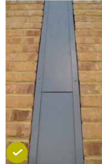
Gas pipes integrated
