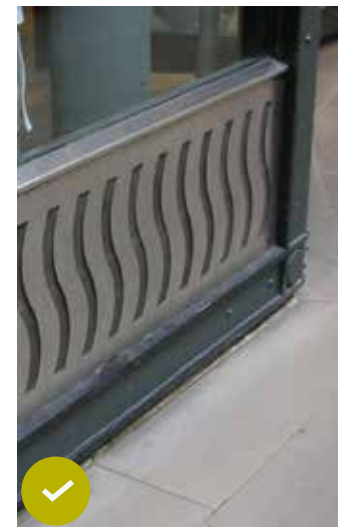
Vents in stall riser
