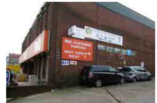
Access to B&Q's car park
