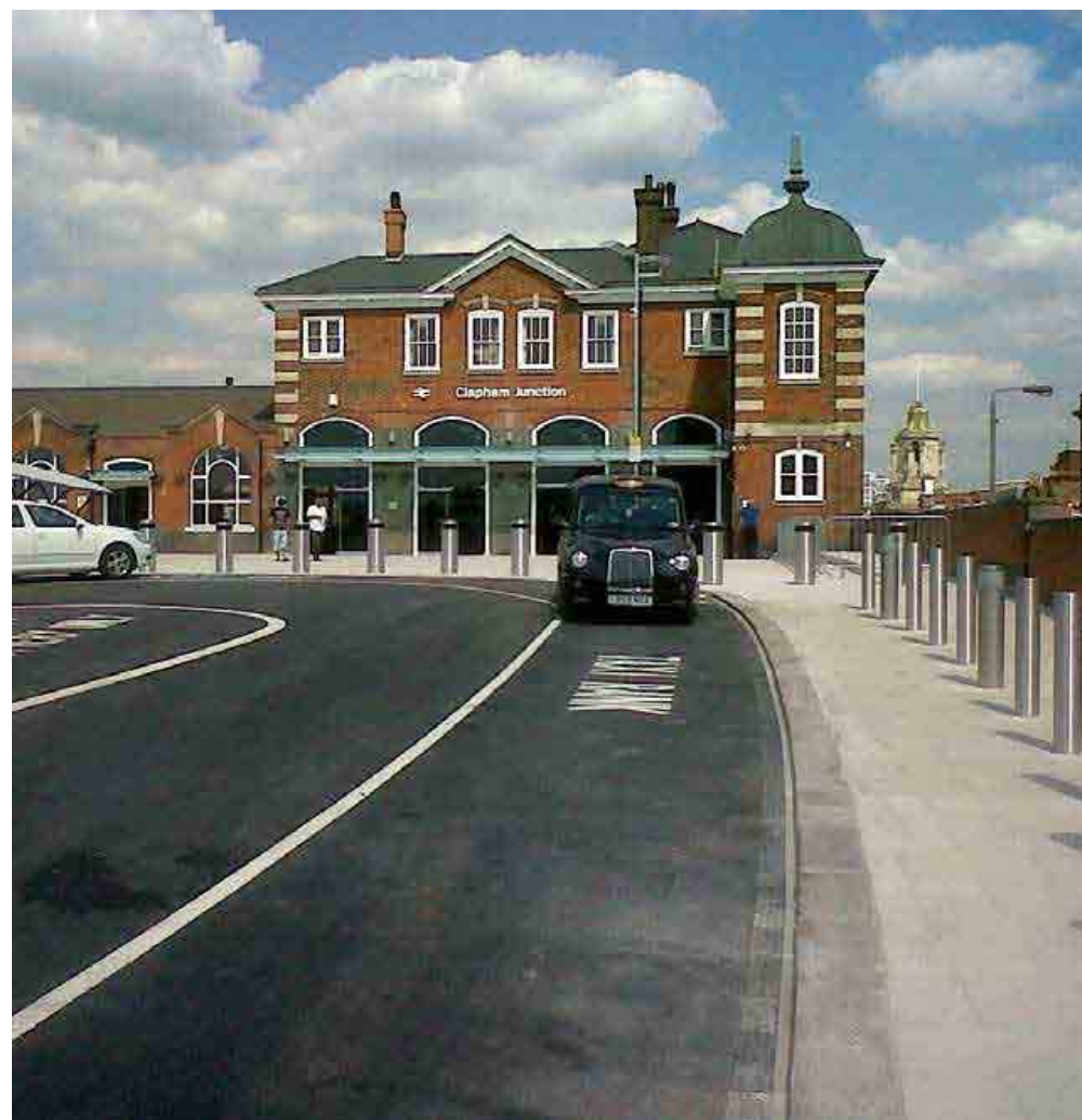
Clapham Junction - Brighton Yard showing an example of redesigned hardscape at Brighton Yard for step-free route into the station from St John's Hill, making it accessible for mobility impaired people and easing congestion in the subway and main entrance
