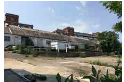
Laundry warehouse and car parking to the rear of Norwood High Street
