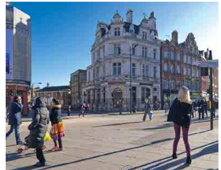
Britannia Junction outside Camden Town tube station improvement scheme significantly improved the safety of pedestrians and cyclists by creating more space with a narrower carriage way.
