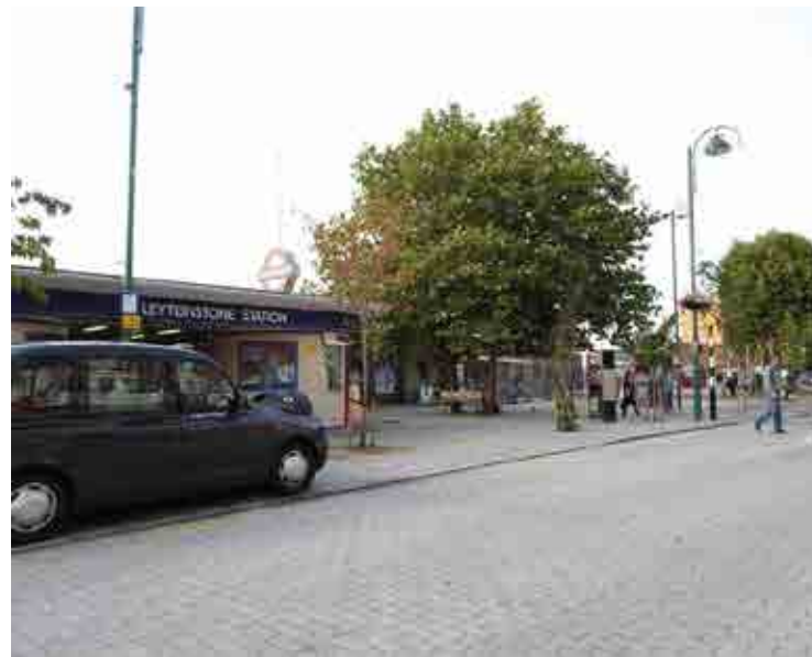
Leytonstone station area, widened footways, realigned pedestrian crossings, improved access to green space, removal of excess street clutter, better signage and more cycle parking spaces.
