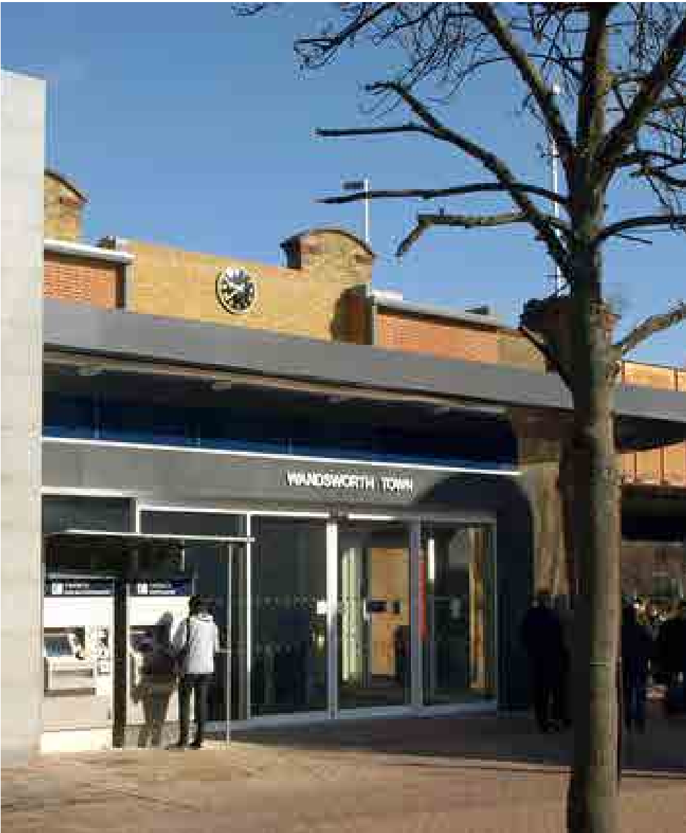
Wandsworth Town station improvements
