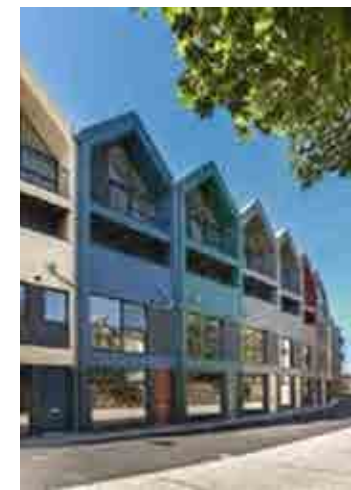
New build live work units at Dragonfly Place in Brockley
