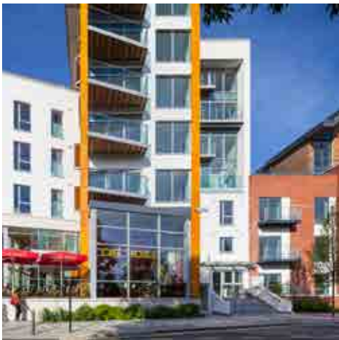
Mixed use development offering new activities and housing in the city centre of Newbury with a focus on community safety and improved sense of place
