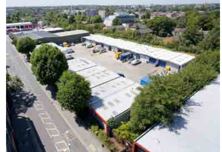
Flexible small industrial units in Herne Hill
