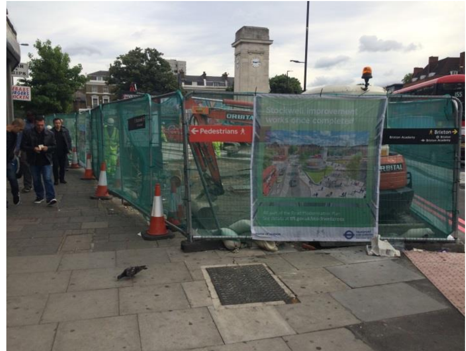
Photo 12.10 Stockwell: Public realm improvements
