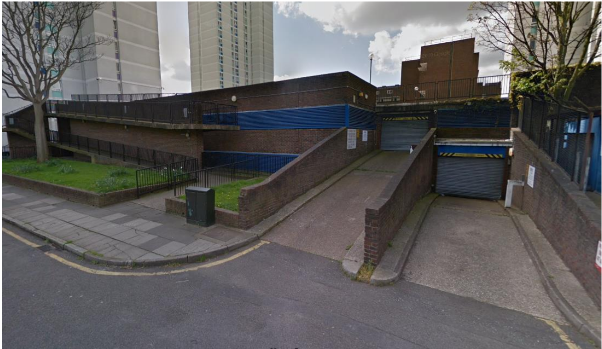
Figure 11 – Part of the Lollard Street development site prior to redevelopment
