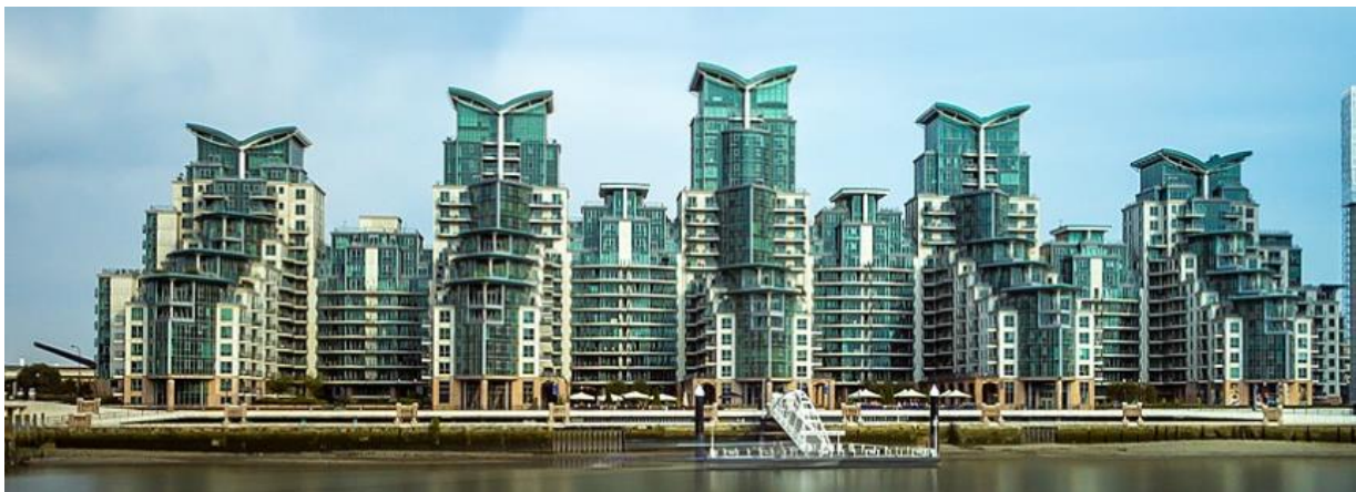
Figure 6 - St George Wharf as viewed from across the River. The highest central part rises to c70m AOD.
