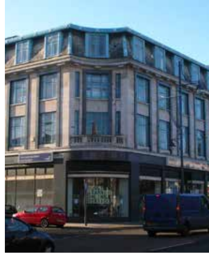
Before additional mansard storey
