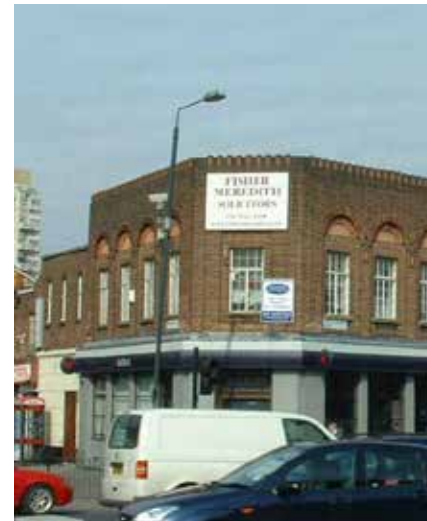
Before additional storey
